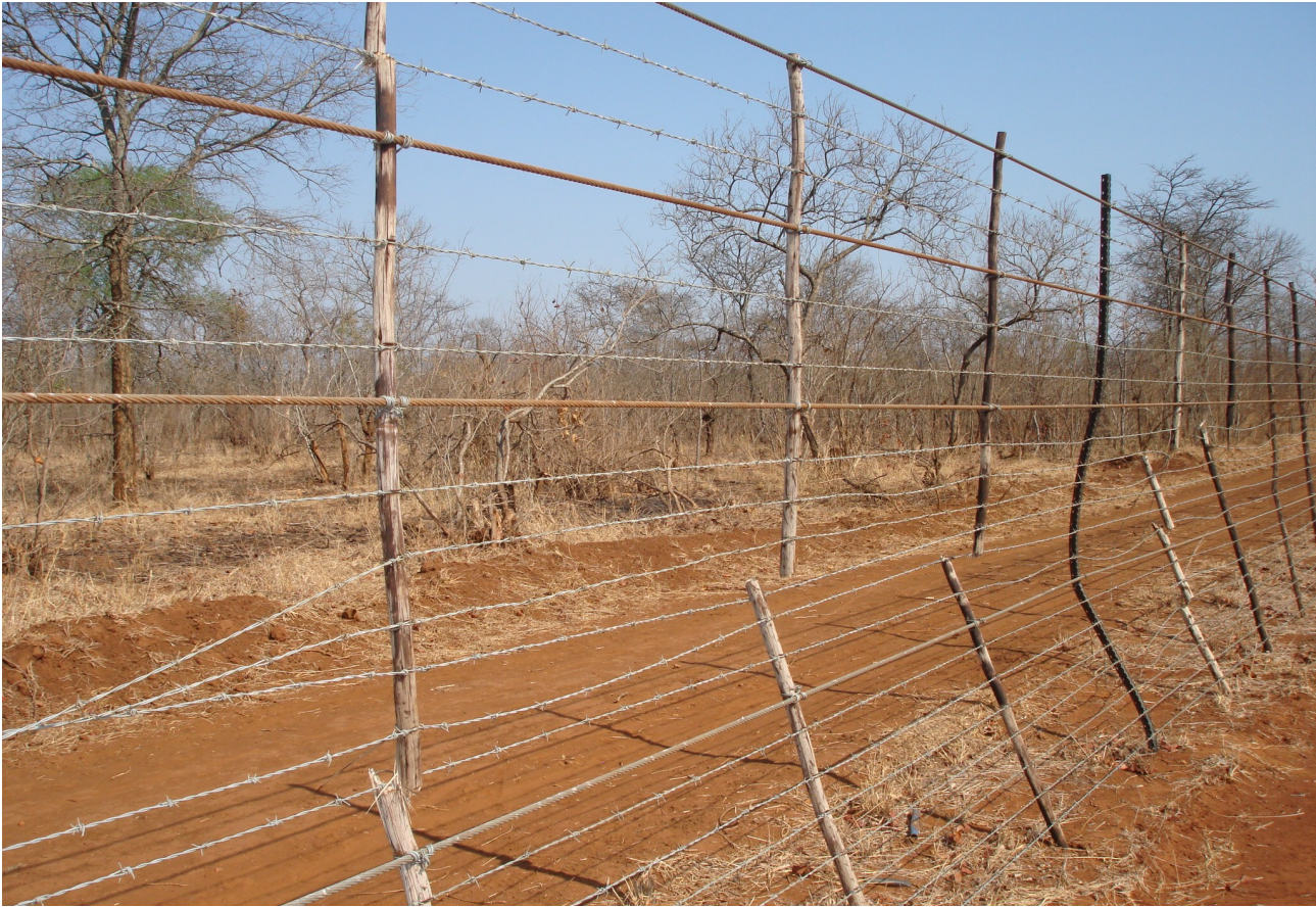
New fencing damaged by elephants at Kruger National Park © Ken Ferguson
